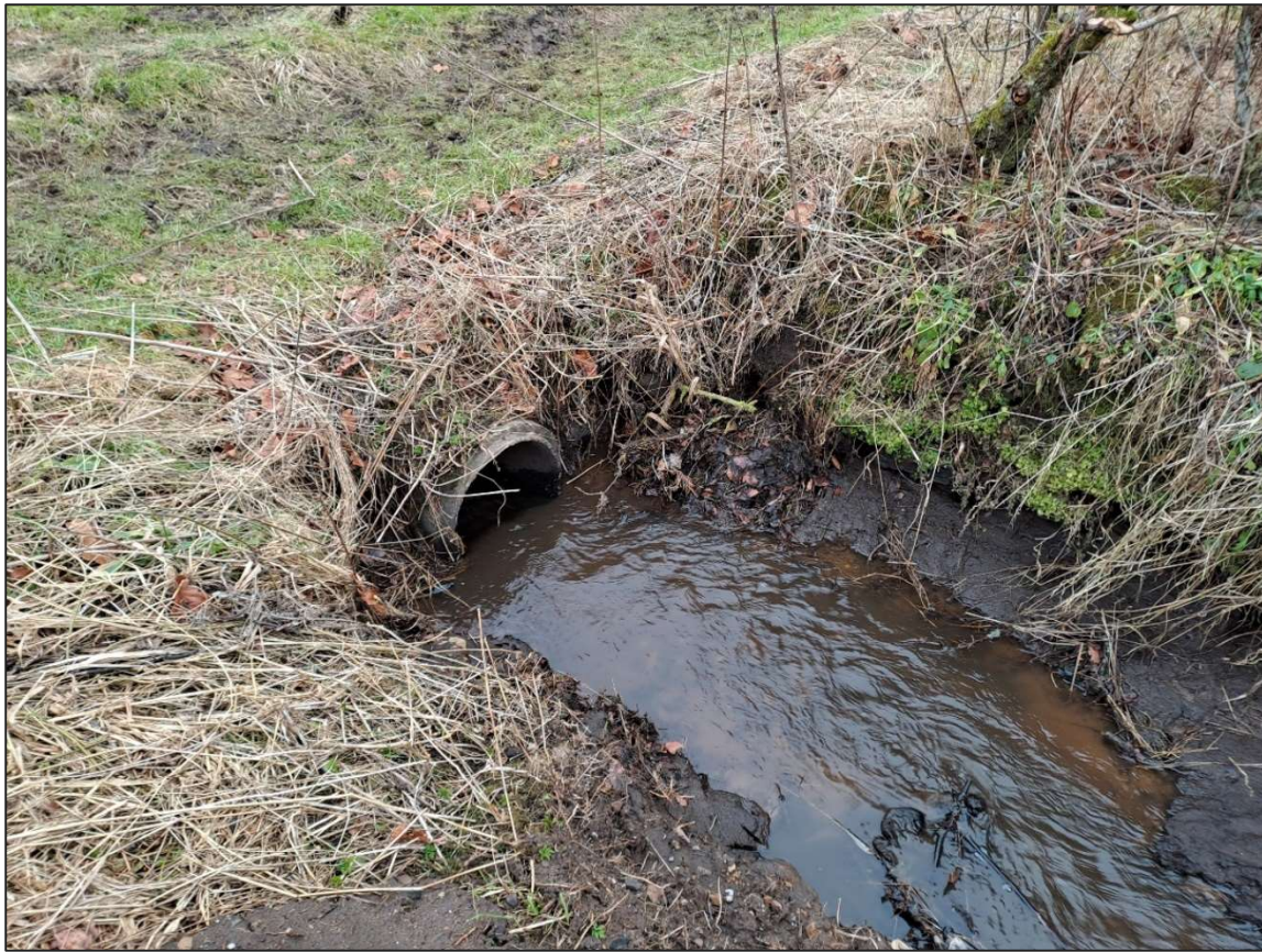
Photograph 1-15 : 450mm culvert under unnamed tributary field crossing
