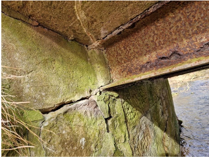
Photo 6 - Cracking Around Steel Embedment
