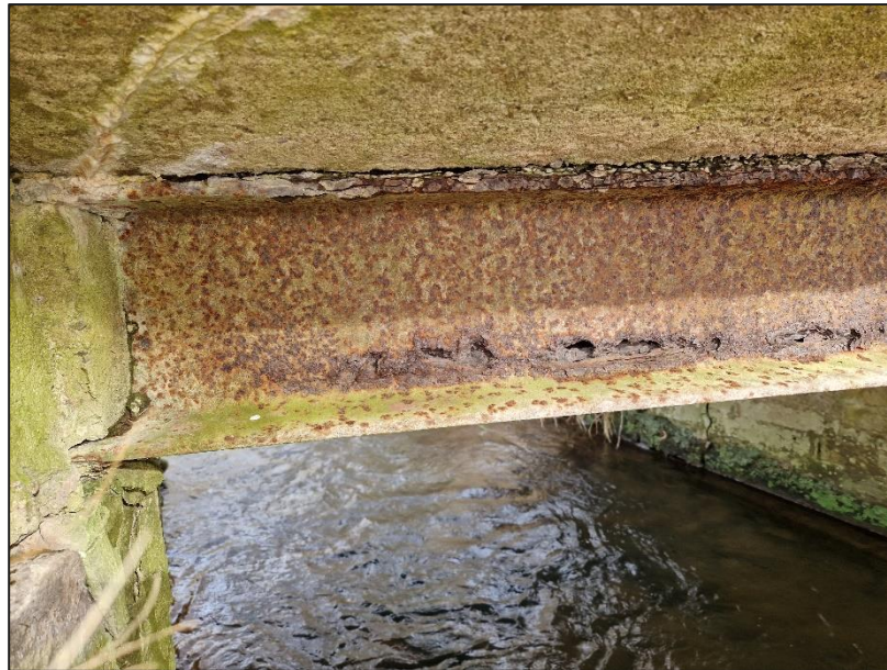
Photo 4 - Steel Beam Corrosion
