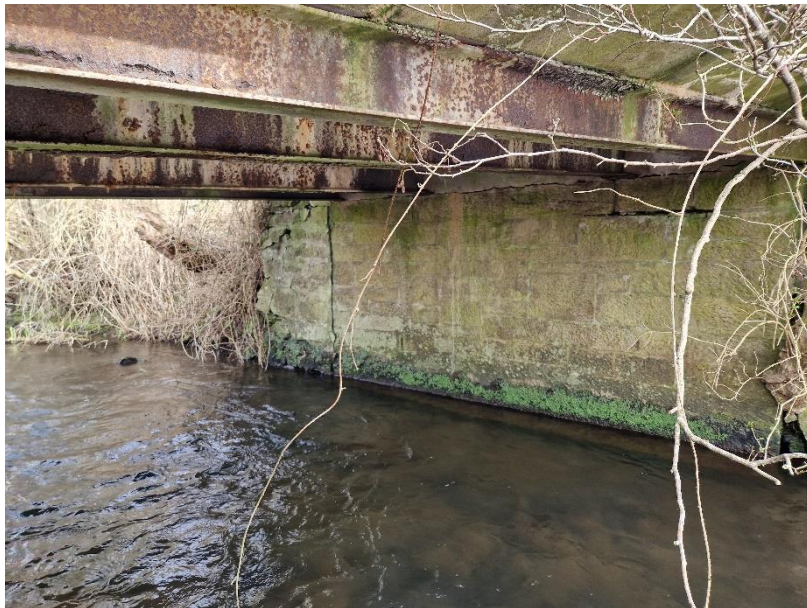
Photo 5 - Abutment Damage
